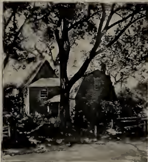
FAIRBANKS HOUSE, Dedham, Mass. Built 1636.
